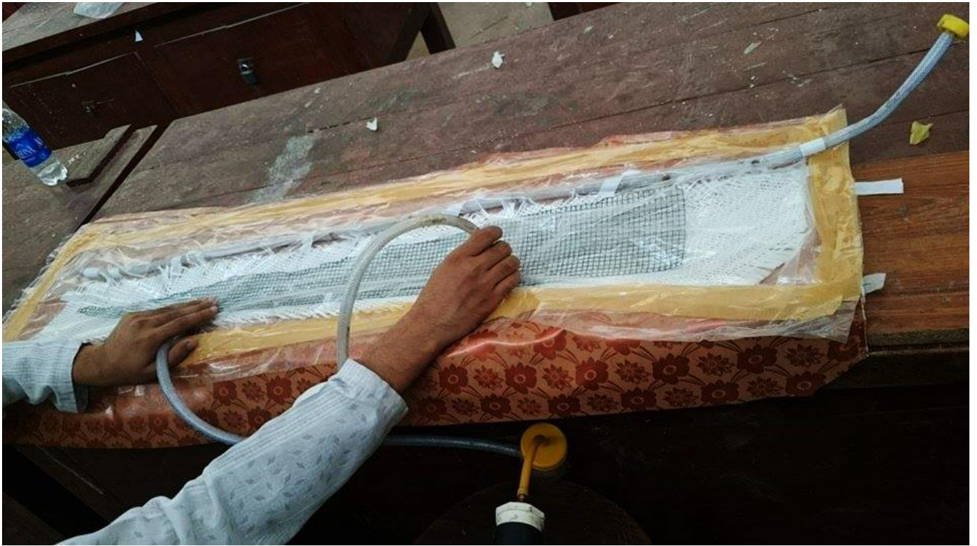
Figure 6. Portable System with Resin Inlet and Suction Points
